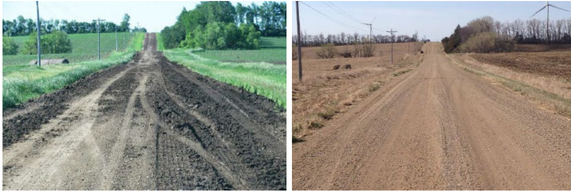
Before/after gravel rehabilitation. Image source: Ken Skorseth, Program Manager, SDLTAP; used with permission
