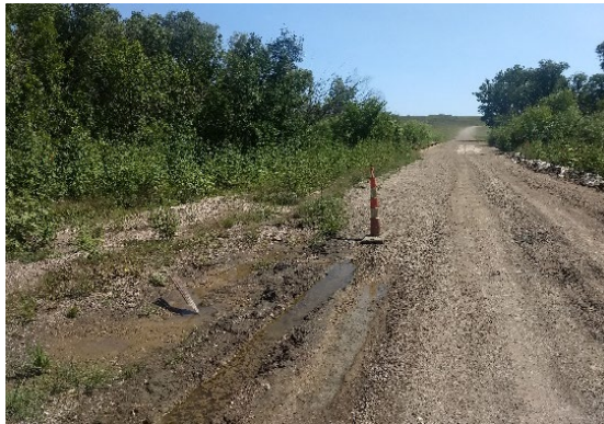
BIA 7 near Virgin Creek Bridge
